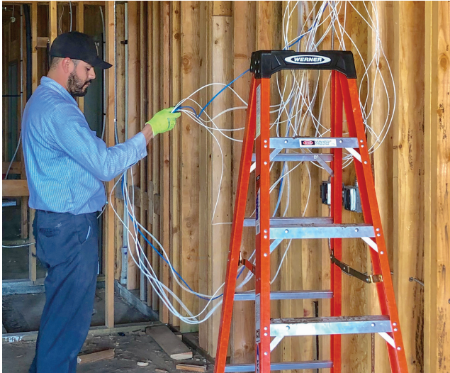
Matson Alarm Company, Inc. custom designs each security system. Shown, installation technician Aaron Rodriguez pulls wire for a commercial project.
